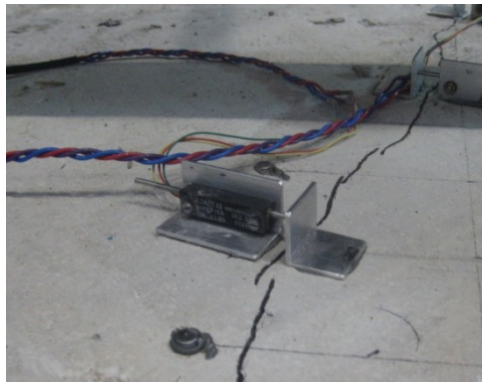
Figure 4.30: Displacement transducer mounted along the crack
