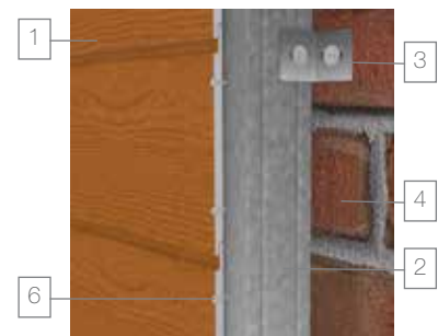
Vertical Fixing Detail
